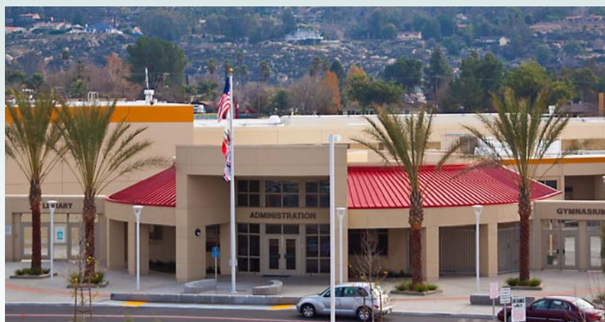
Hemet High Renovation Project—Admin Bldg 2011
